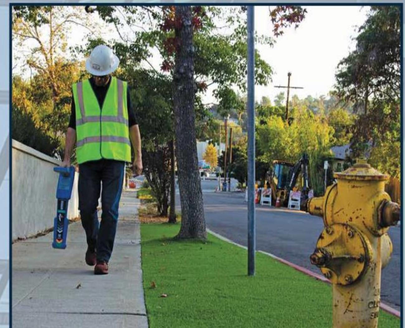
Pipes with Cathodic Protection System can be followed using the CPS passive mode. CPS compass mode ensures alignment with the target pipeline.
